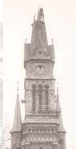
Blown up tower, 1956
